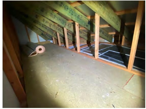
Storage void over patio
