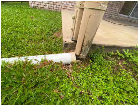
Downpipe leaking
